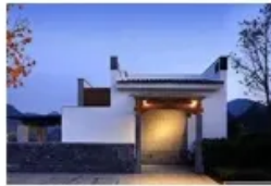
Household Energy Storage
