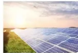
Energy Storage System
